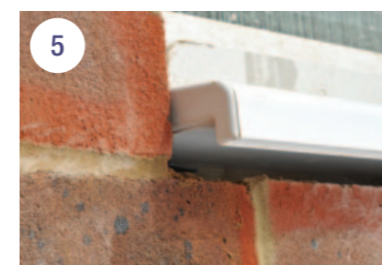
Movement gap under window
