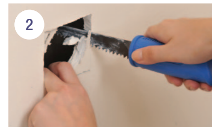
2 Drill holes to get started then cut with a pawsaw
