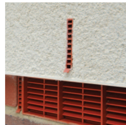
Cavity vents ensure the timber frame is kept dry. Here, the large vent is for a suspended timber ground floor.
