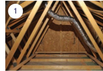
OSB sheathing on the gable wall
