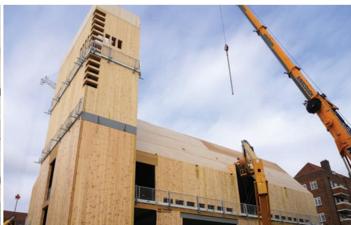
**Image 3 - Multi storey CLT frame**
